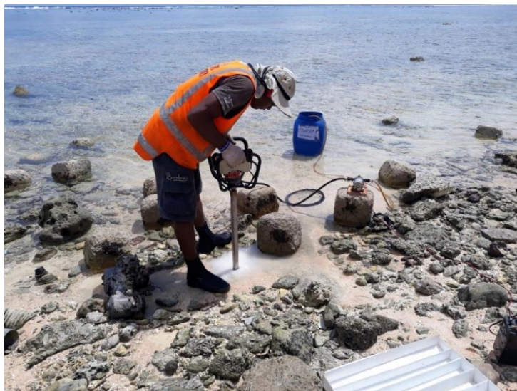
Figure 6: Rotary coring using the Shaw Portable Drill.
